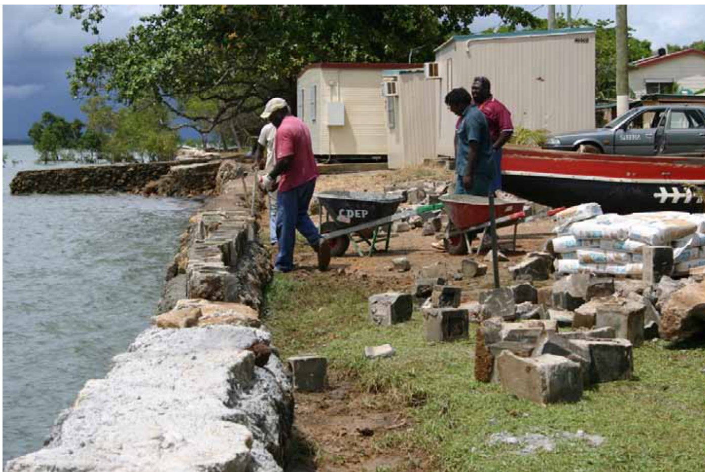
Rebuilding the sea wall
